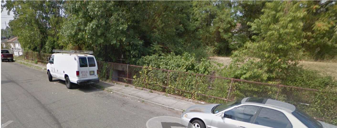
Tunnel Existing Conditions (View from Catherine Street facing tunnel)
